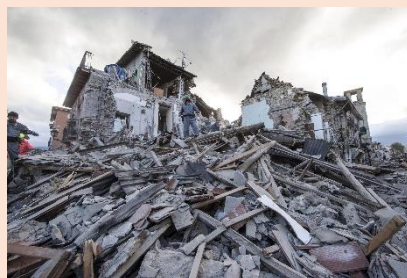
Damage to structure
