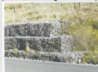
Figure 1 Gabions along the side of a road
